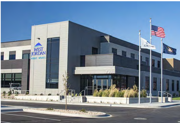
West Jordan Public Works Building 7960 South 4000 West
